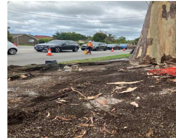
Centre Dandenong Road, Cheltenham – footpath reconstruction during construction
