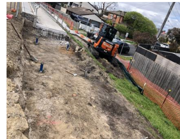
Dahmen Street, Carrum – ramp during construction
