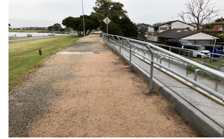
Dahmen Street, Carrum – ramp after construction
