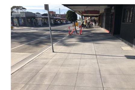
Como Parade West, Mentone Shopping Centre – west side footpath replacement after construction
