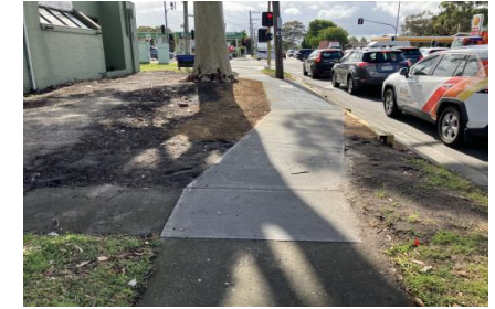
Centre Dandenong Road, Cheltenham – footpath reconstruction after construction
