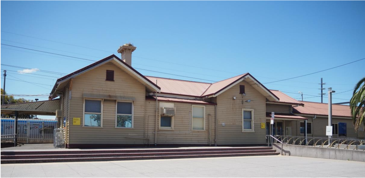
Mordialloc Railway Station (HO91). (Source: RBA November 2022)
