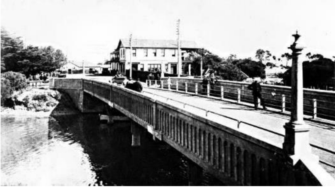
Concrete Mordialloc Bridge, 1920s. (Source: Mordialloc and District Historical Society)
