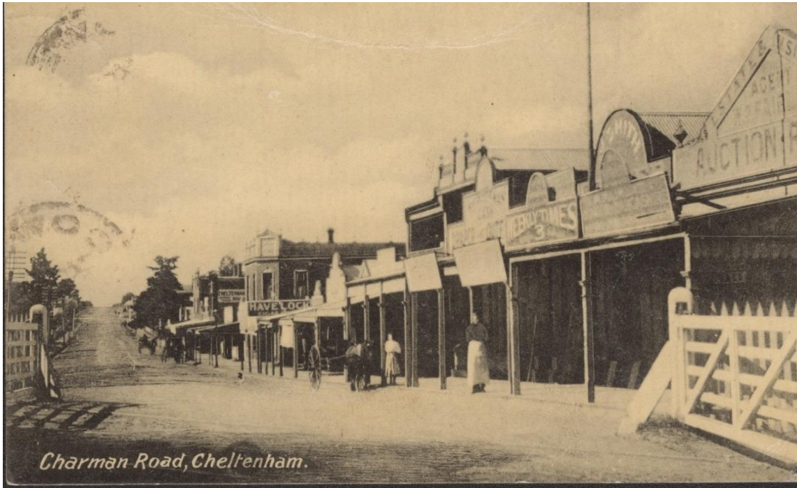
Shops along Charman Road, Cheltenham, 1915 (Source: SLV, H90.140/37)
