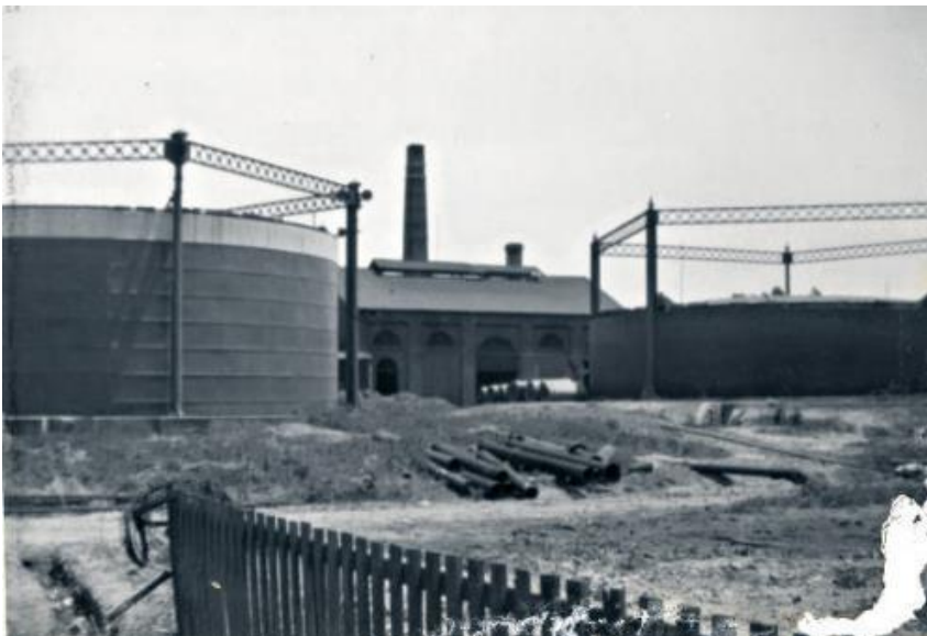
The Mentone gas works, located on Brindisi Street, 1928. (Source: Mordialloc and District Historical Society)
