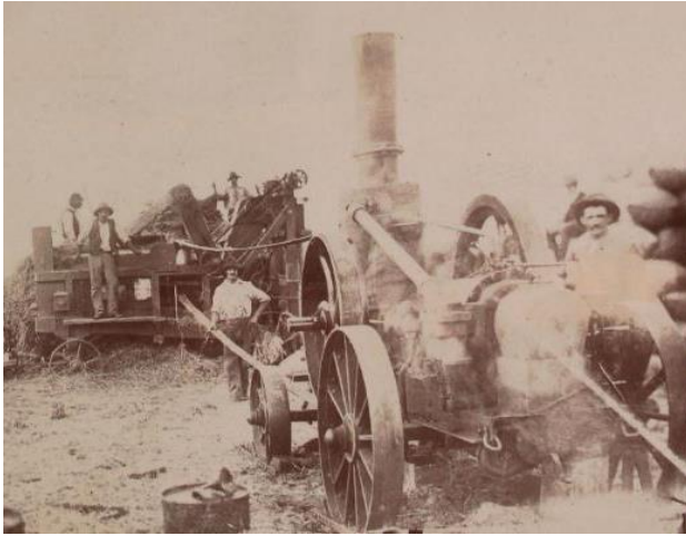
Early machinery used at Carrum, 1903. (Source: Roland Bishop, SLV)
