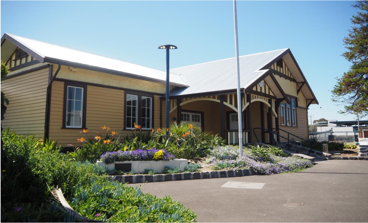
Mentone Railway Station and Gardens (HO106). (Source: RBA, November 2022)
