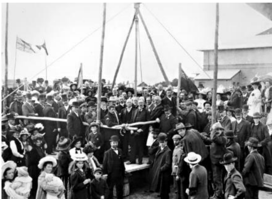
Laying of the foundation stone for Benevolent Asylum at Heatherton, 1909. (Source: Kingston Collections, City of Kingston Library)
