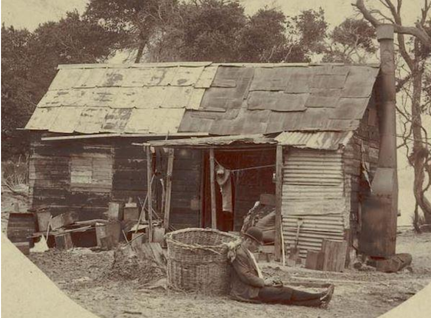
Early dwellings – the McLean family cottage, Mentone, circa 1905. Demolished. (Source: Museums Victoria)
