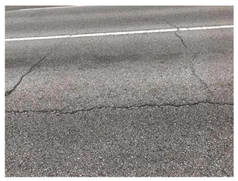
Sections 4— Mcindoe Pde to Bay Street — Approximate length of the section is 400 m. This section of road is in satisfactory condition and has a condition rating of 5. Longitudinal cracks have appeared and needs crack sealing. Estimated life of this section could be 4 to 6 years. (Approximately half of this section is not within the current contract length i.e. 200m approx.).
