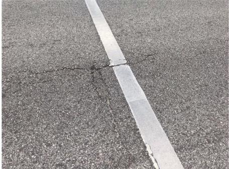
\*\*\*Sections 3—Parkers Road to Mcindoe Pde- This 300m section of road is in poor condition and has a condition rating of 6. Areas of pavement exhibit significant cracking and needs patching work soon. Estimated life of this section could be 2 to 4years. (Checking of aerial photos indicates that this section has not been resurfaced in at least 10 years).
