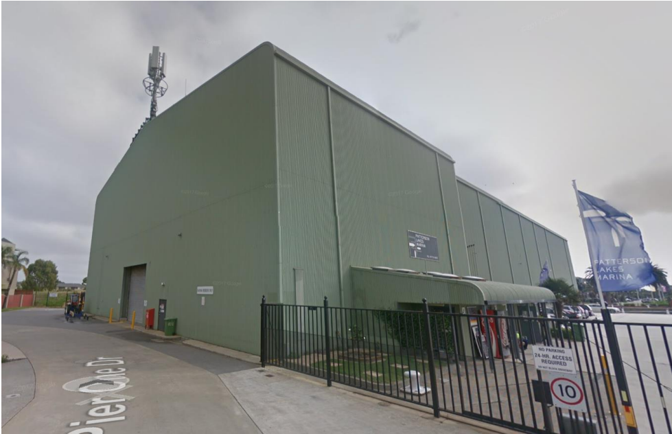
Site 2 viewed from Pier One Drive:
