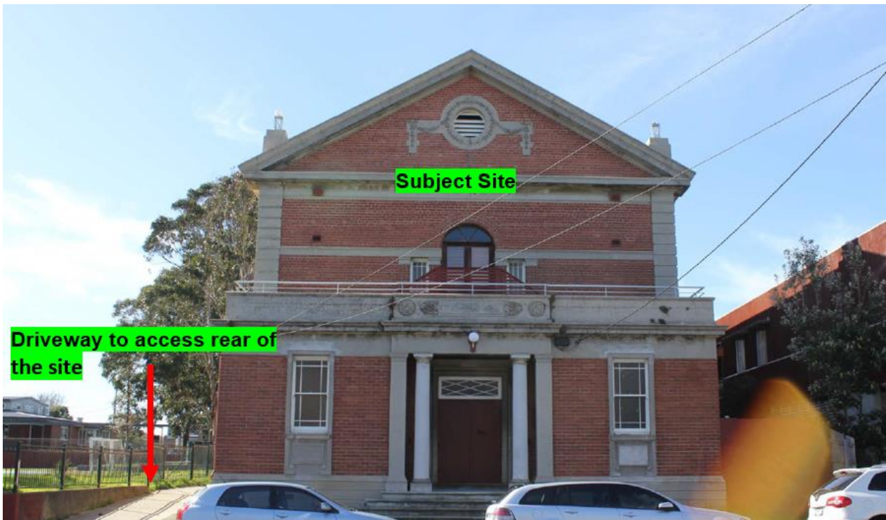
Looking north east at subject site from street frontage.
