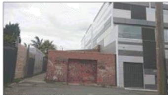
VIEW OF SUBJECT SITE FROM FAIRVIEW LANE
