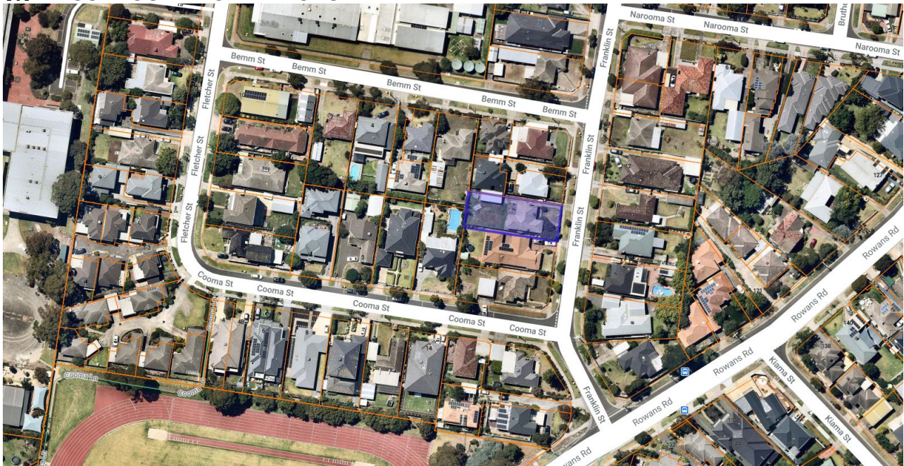
Image 2: Aerial view of subject site
