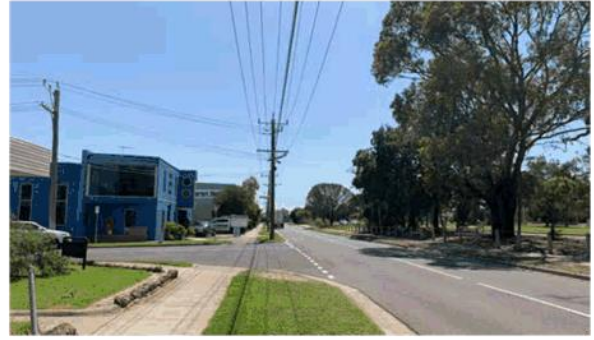
View along Linton Street, looking north. The large format warehouse retail presents an inactive frontage to the street.
