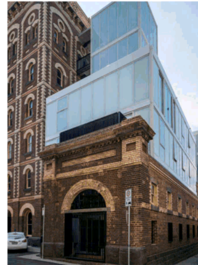
Figure 35: Yorkshire Brewery Residential Complex - Collingwood VIC
