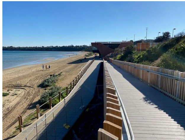
Figure 14: A new ramp leading down to Mentone beach in Kingston.
