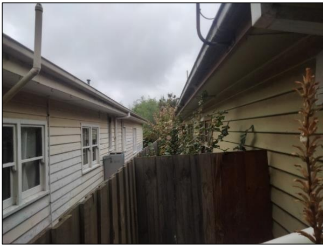
Eastern boundary viewed from north
