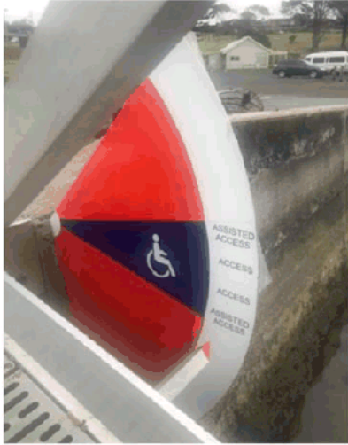
Figure 6-1: Gangway gradient gauge at Hopkins in Warrnambool Shire, Vic
