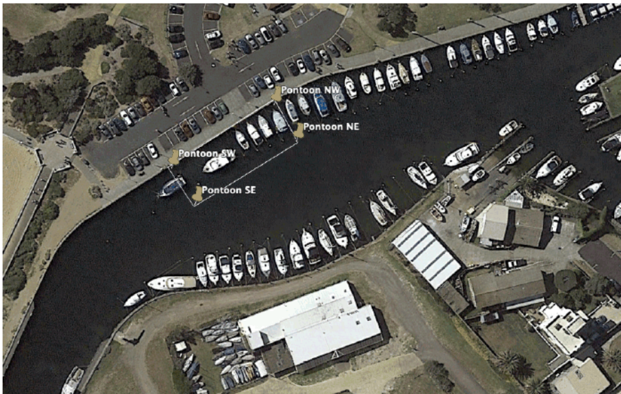
Figure 1 Mordialloc Creek Accessible Pontoon location (reference Google Earth pro).
