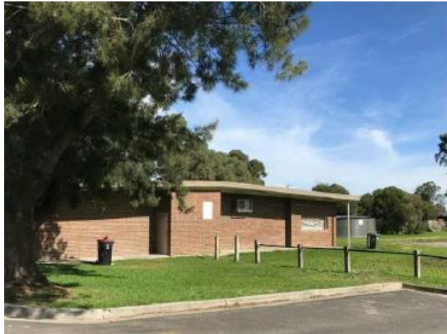
Existing pavilion to be demolished
