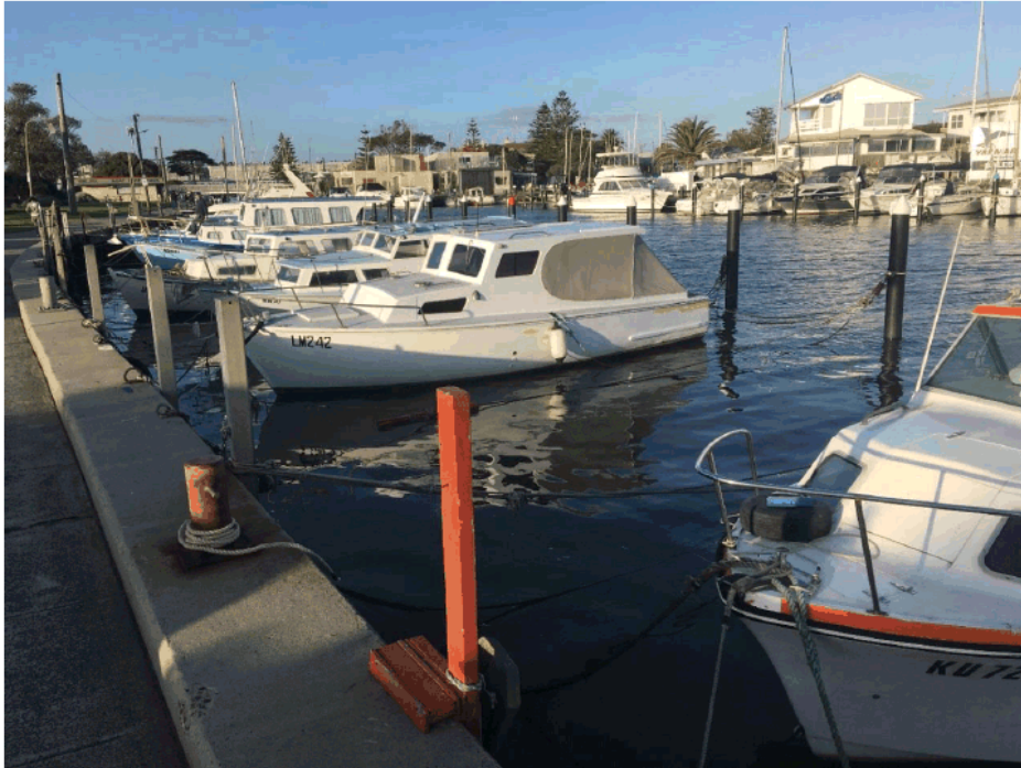
Figure 6: Site Photograph (4 June 2020)
