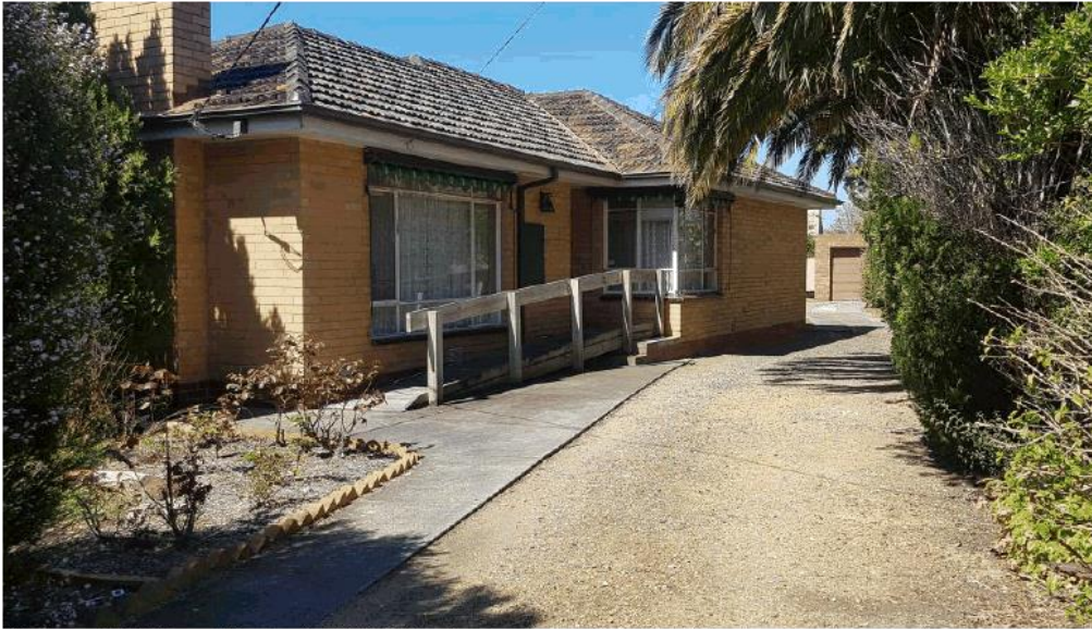
Photograph 1: View of the front of 66 Golden Avenue from within the driveway
