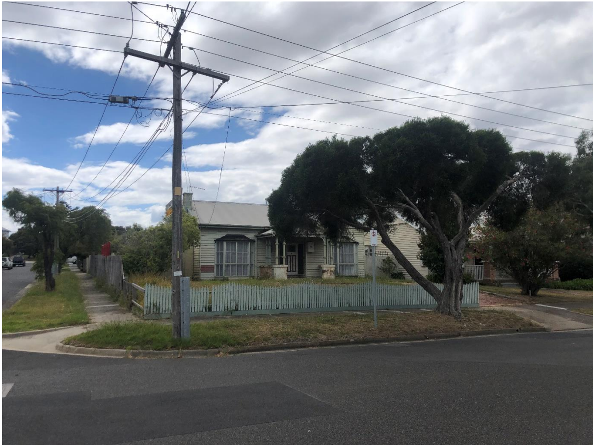
Image 1: View looking north towards the Powlett Street frontage of the site (1 March 2021).
