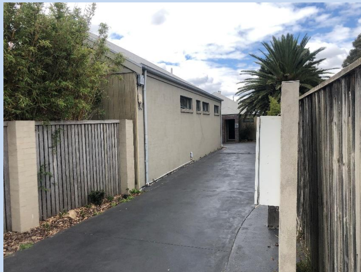
Image 3: View, looking east, of the driveway to the rear dwelling and the highlight windows of the front dwelling (1 March 2021).
