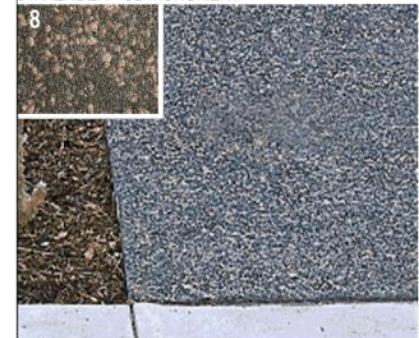
08. DRIVEWAY - EXPOSED AGREGATE
