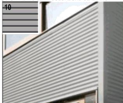
10. METAL HORIZONTAL COLORBOND CLADDING
